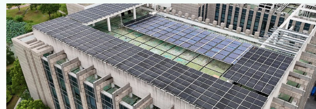
Rooftop photovoltaic module array at the Fangshan Park of BOC Jiangsu Branch.
