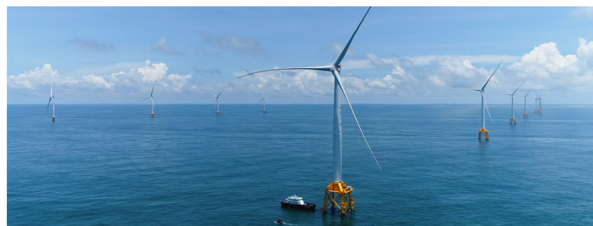
BOC Guangdong Branch supports the construction of an offshore wind farm at a port.
