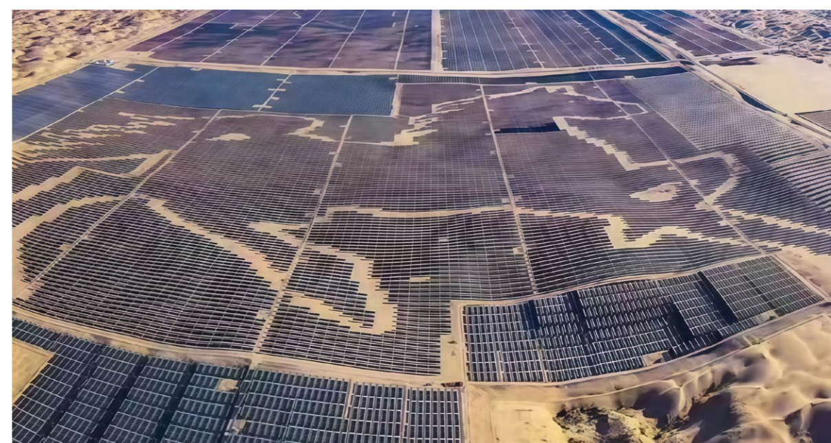
Inner Mongolia Branch provided fixed asset loan support for the photovoltaic "Top Runner" Base Project in Dalad Banner, Ordos City.
